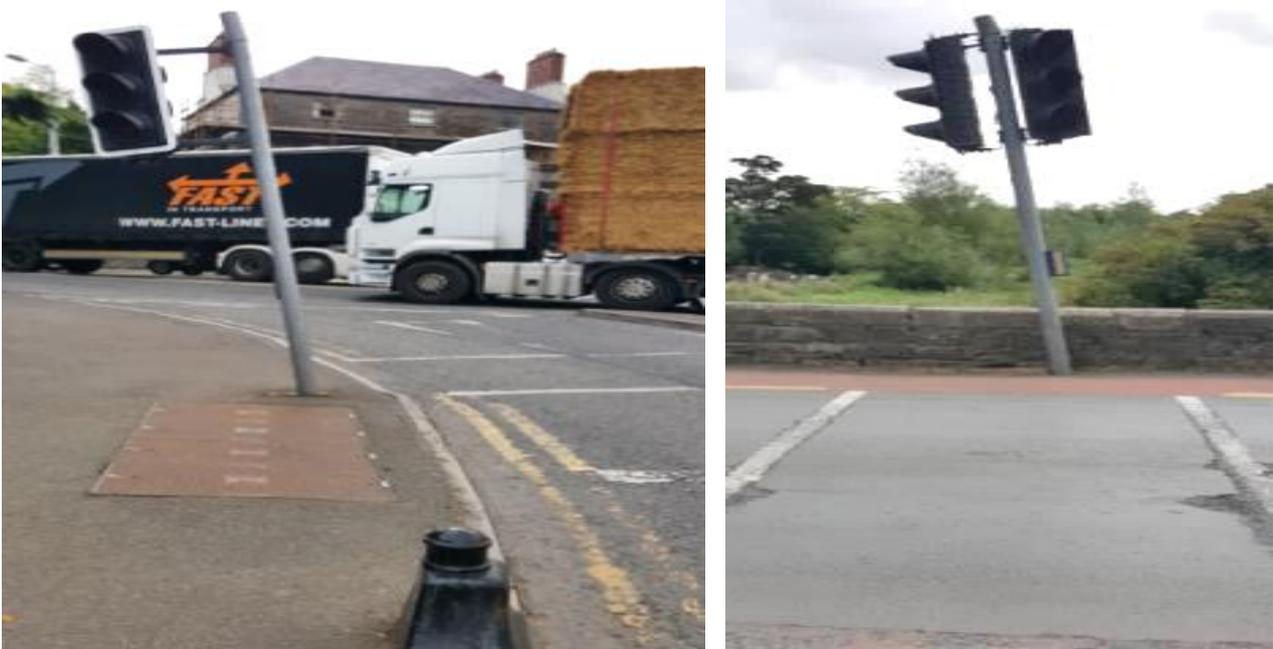
**Figure 2.11: Examples Showing Damage to Traffic Signals at The Square and Slane Bridge**
